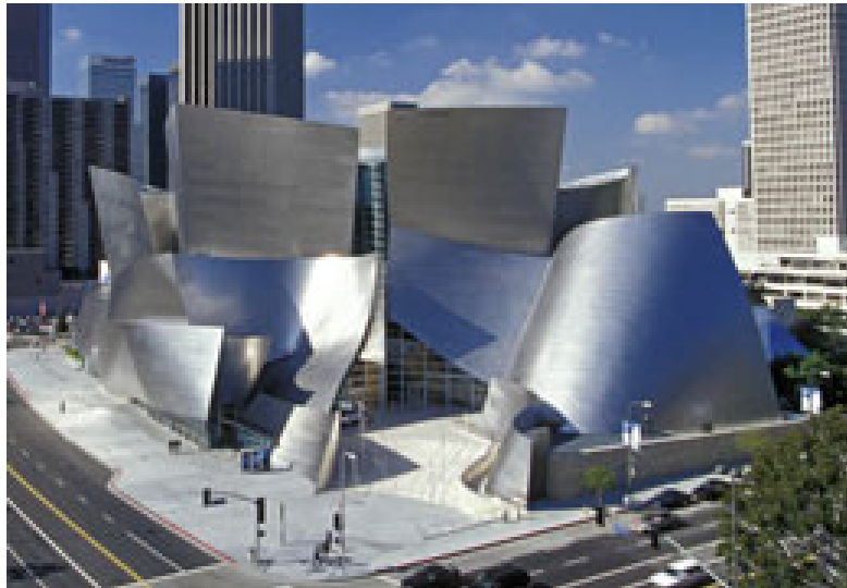
Figure 4 Walt Disney Concert Hall, Los Angeles (2003) Photo credit: Michael L. Magat from "DIGITAL PROJECT - Frank Gehry's vision" March 9th - May 20th 2007.
